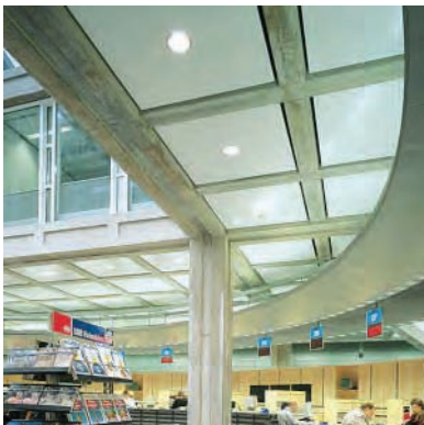
Barcol-Air radiant ceiling technology, cassettes and circular segment panels
