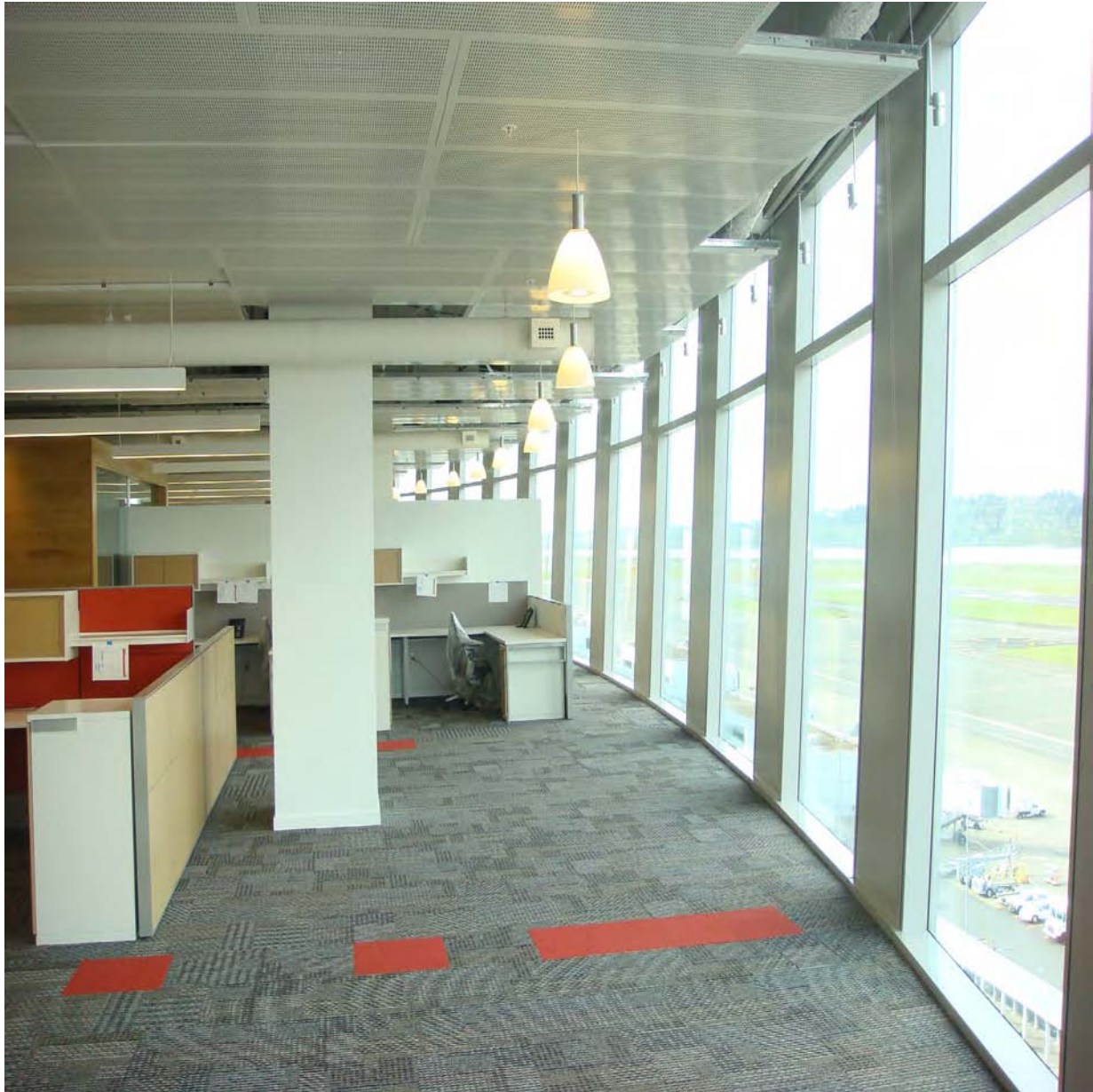
BRC chilled ceilings and rectangular panels
