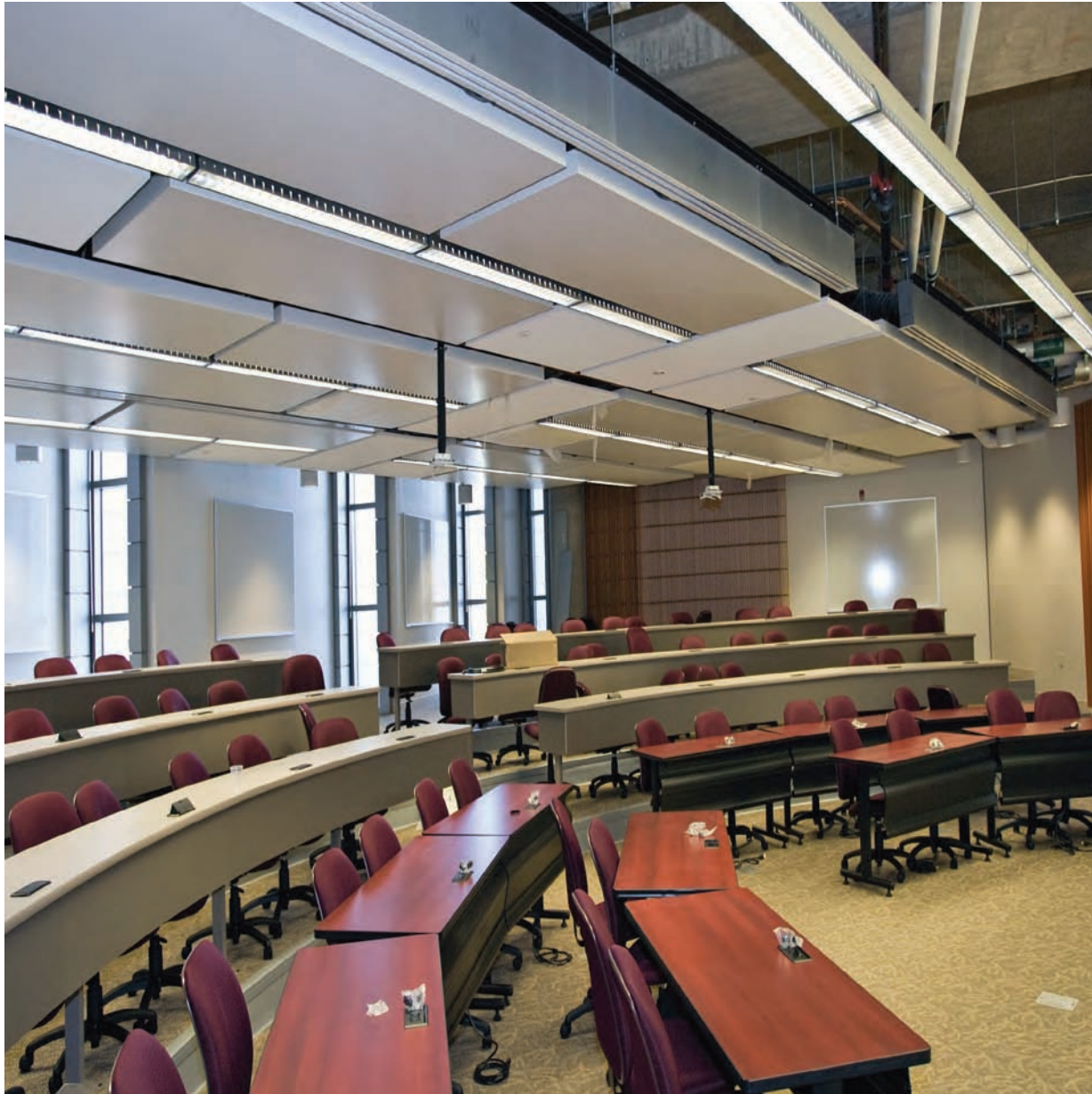
Space cooling with Barcol-Air radiant ceilings
