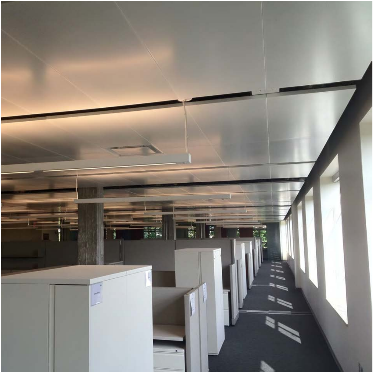
Barcol-Air radiant ceilings in offices
