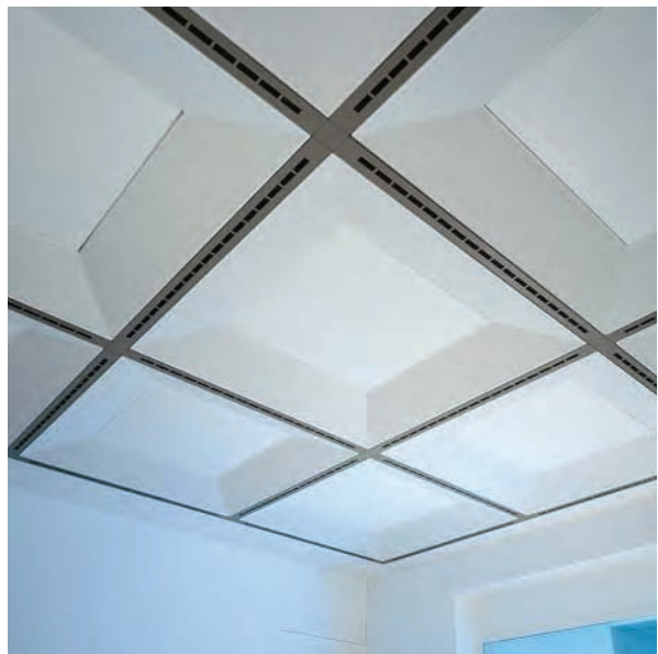
BRC chilled ceilings in cassette form
