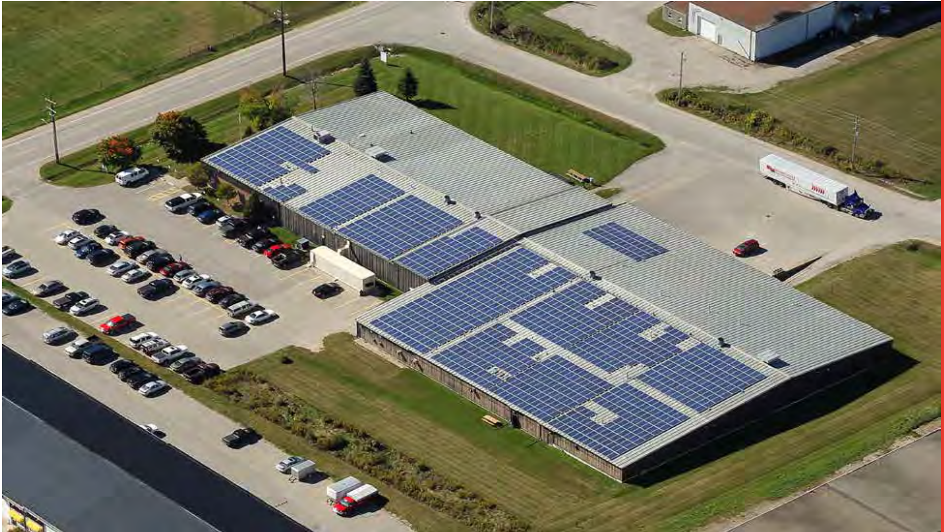
CGC Group Manufacturing Facility in Fergus, Ontario, Canada (Solar PV panels on roof)
